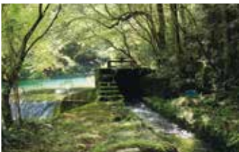
毎床溝の取水堰
